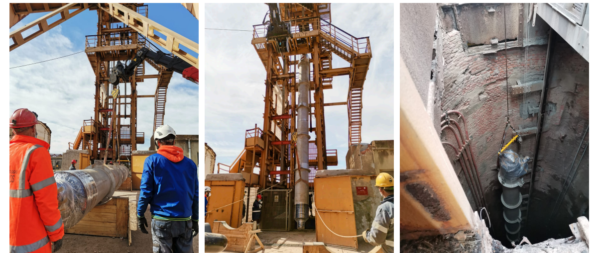
Test installation of the module
