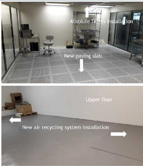
Figure 2: LMA ISO3 clean room area that will be modified. top : area where the new profilometer will be installed. bottom : on the upper floor, location of the future clean air station
